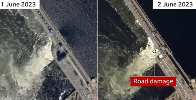
Satellite images show damage to roadway
